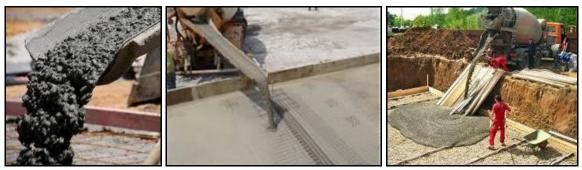
Photograph 6. Photos showing SCC discharging through truck via chute
