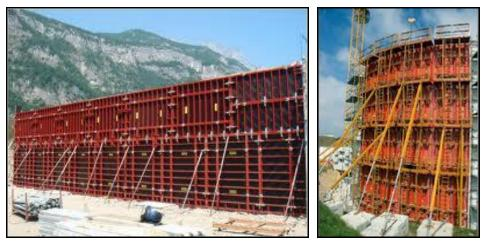
Photograph 4 Formwork erected for SCC
