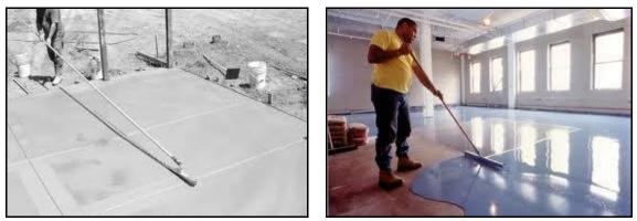
Photograph 8. Leveling SCC with a skip float
