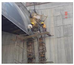
Photograph 7. Photos showing Placing of SCC by skip
