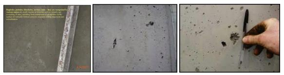
Photograph 10. Photos showing the bugholes on concrete surface.
