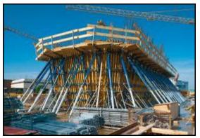
Photograph 5 Formwork erected for pumping SCC bottom up
