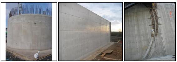
Photograph 9. Photos showing finished surface of SCC
