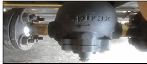
AFTER-FLOAT TYPE TRAP
