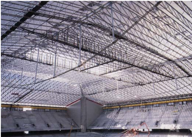
The 65,000-seat multi-purpose Alamo Dome, San Antonio, Texas 408,800 ft 2 NA G90 Painted White.
