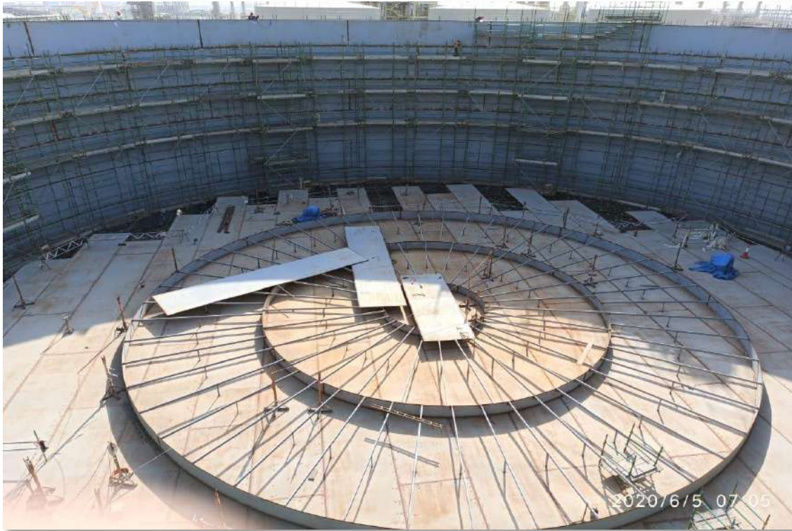
BAPCO – BMP PROJECT , BAHRAIN (STORAGE TANK) - CONSTRUCTION OF DOUBLE DECK
