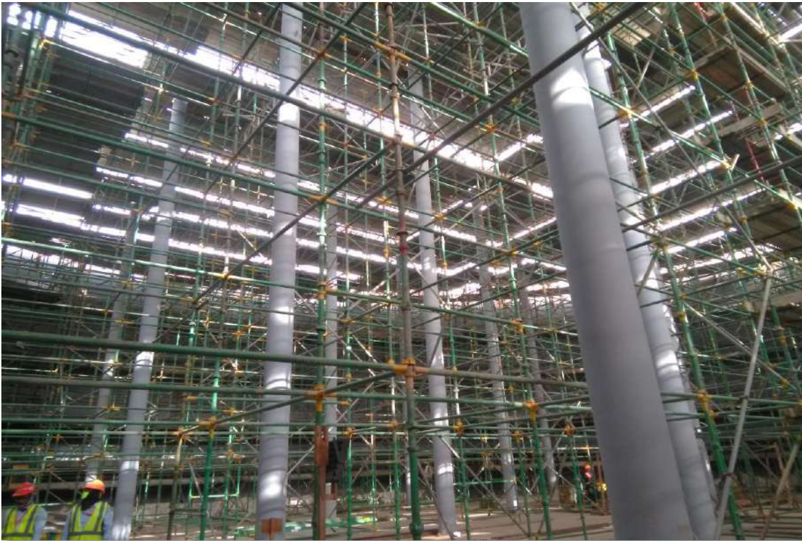
BAPCO – BMP PROJECT , BAHRAIN (STORAGE TANK) - COLUMN SUPPORTED CR TANK
