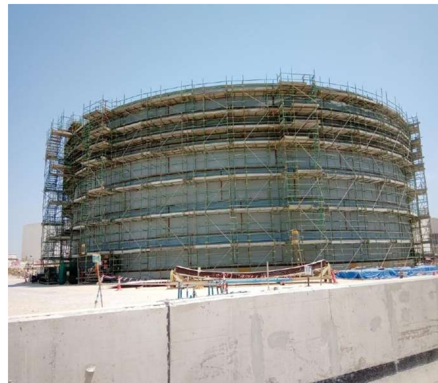
BAPCO – BMP PROJECT , BAHRAIN (STORAGE TANK) – DOUBLE DECK EFR TANK
