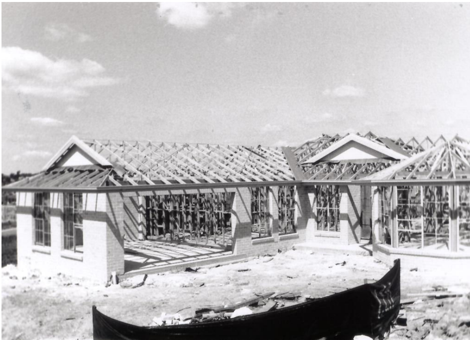
Fig. 95 The completed roof frame
