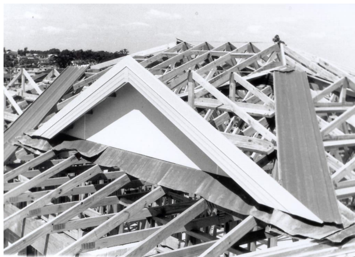
Fig. 93 Prepared trussed roof ready for tiles
