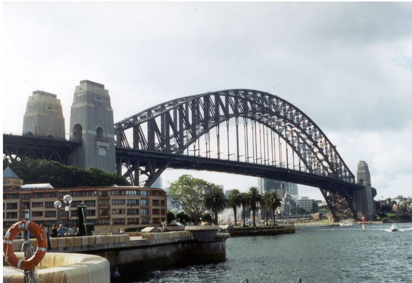
Fig. 7 A well known trussed structure - Sydney Harbour Bridge
