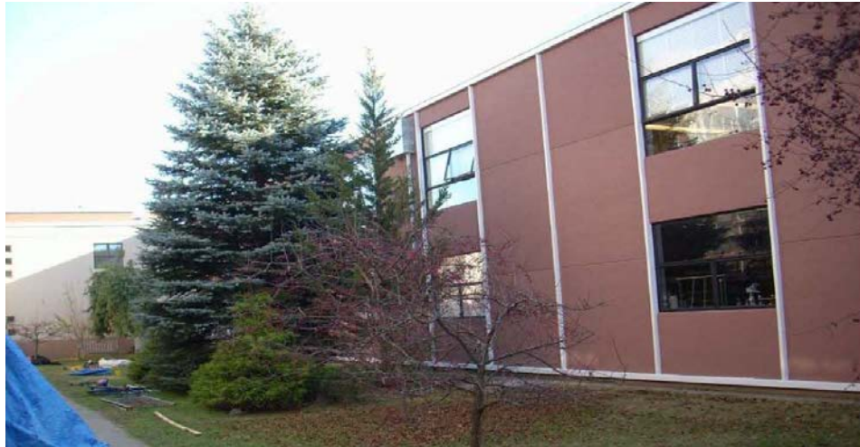
Figure 3: The finished project; an insulation value of R-10 was added.
