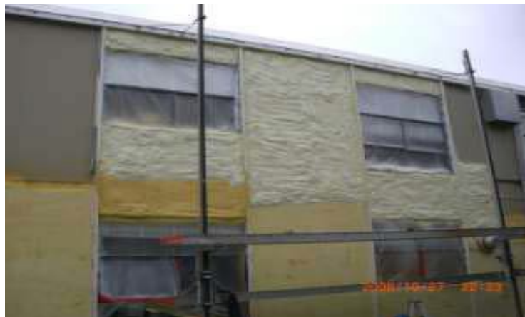
Figure 1: High school in Vermont, Application of SPF (top) shown before and after trimming (bottom).
