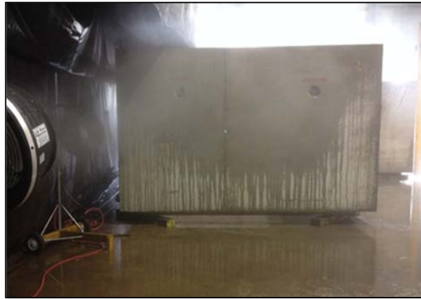
Fig. 36: Temperature & Moisture Control During Steam Curing
