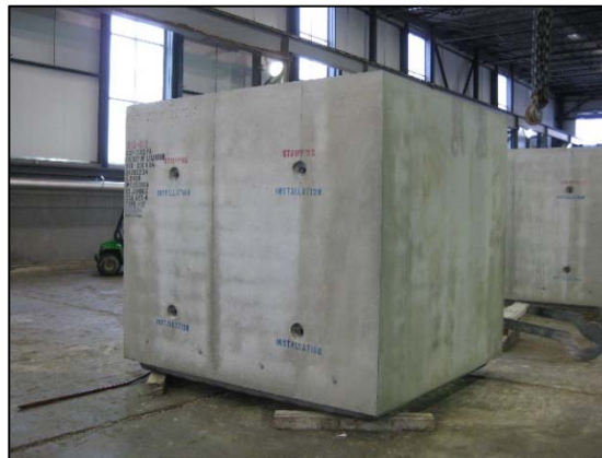
Fig. 32: Wet Cast Box Stripped After Curing
