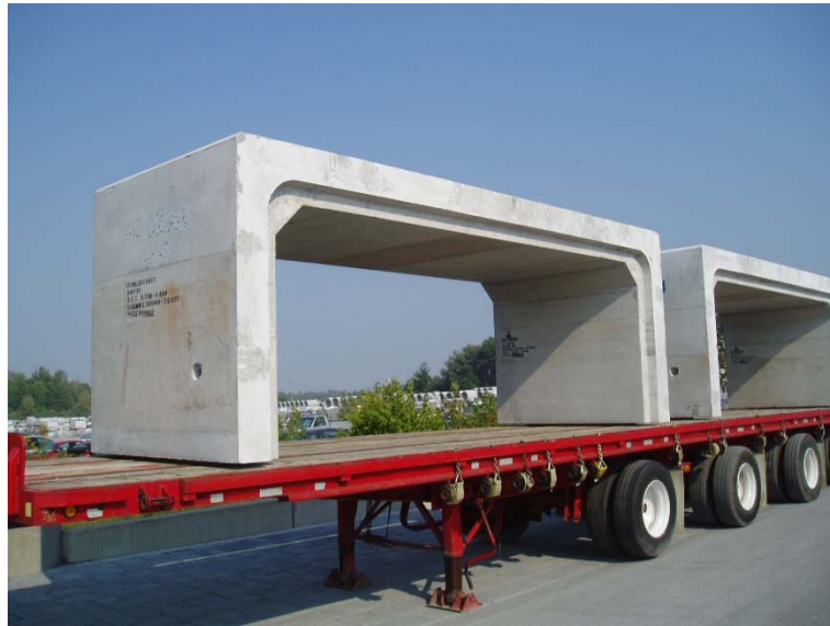
Fig. 5: Check Shippable Limits for Precast Products
