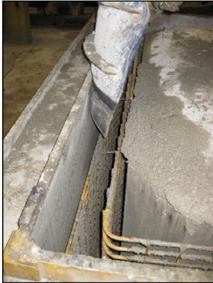
Fig. 33: Filling Dry Cast Box Form
