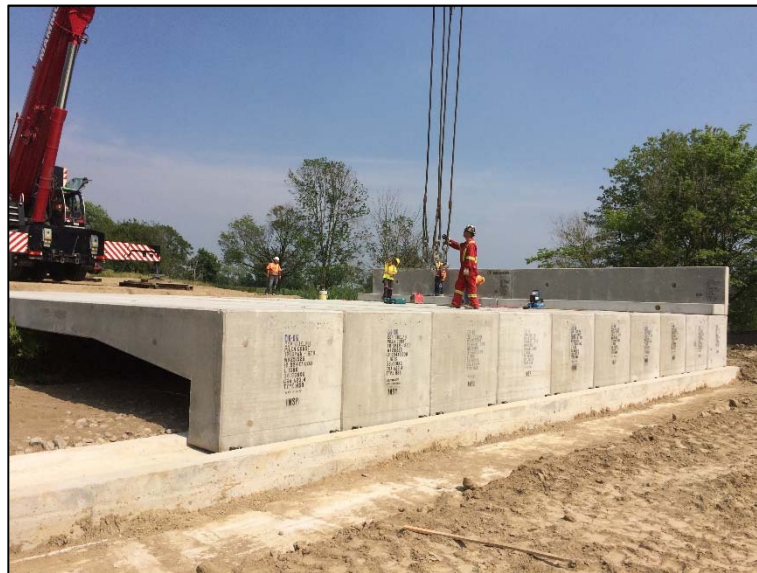
Fig. 7: Open Profile Box Installed on Footings
