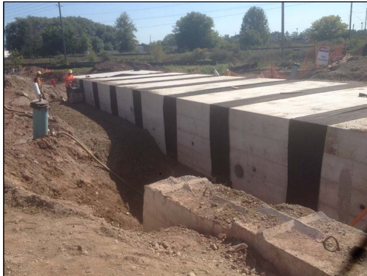
Fig. 48: Backfilling the Culvert
