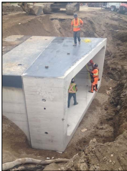
Fig. 15: Skew End Unit for Culvert
