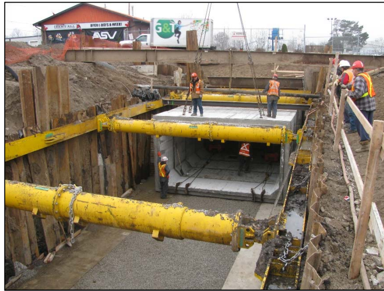
Fig. 39: Box Puller Used for Box Unit Installation
