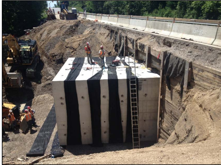
Fig. 43: Filter Fabric Wrapped Over Joints
