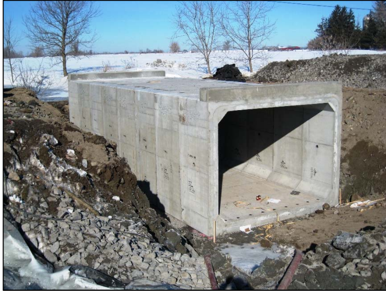
Fig. 17: Culvert with Precast Header Walls
