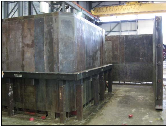
Fig. 30: Modular Formwork to Assemble
