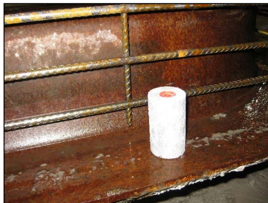
Fig. 25: Chair to Keep Cage Off Pallet
