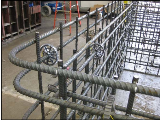
Fig. 26: Fabricated Rebar Cage
