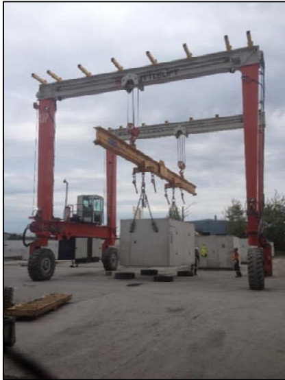
Fig. 45: Lifting with Spreader Beam
