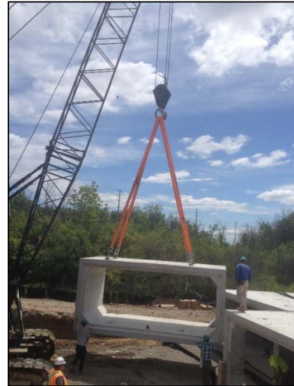
Fig. 46: Lifting with Lifting Straps
