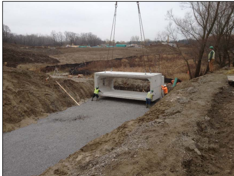
Fig. 3: Constructed Foundation for Boxes
