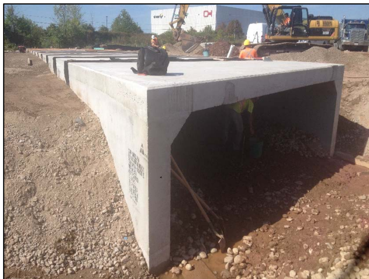
Fig. 49: Backfilling Complete Along Culvert Sides
