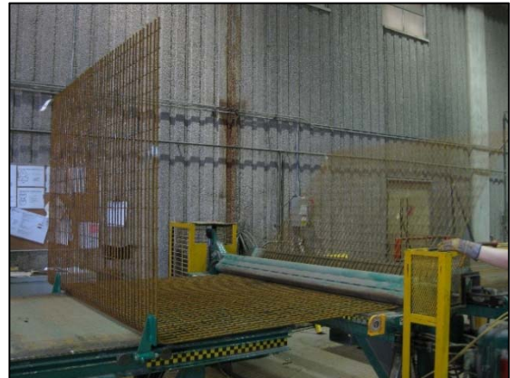
Fig. 21: Bending WWR Mats
