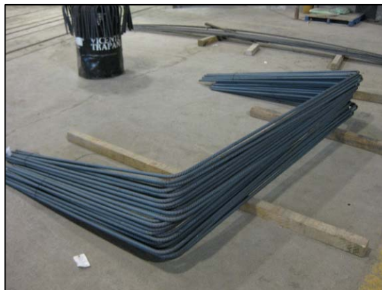
Fig. 22: Rebar Bent for Cage Construction
