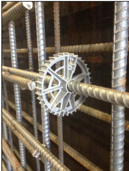
Fig. 28: Plastic Wheel Spacer
