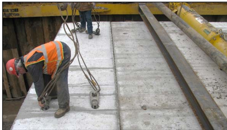
Fig. 44: Lifting Anchors in Top Slab of Box
