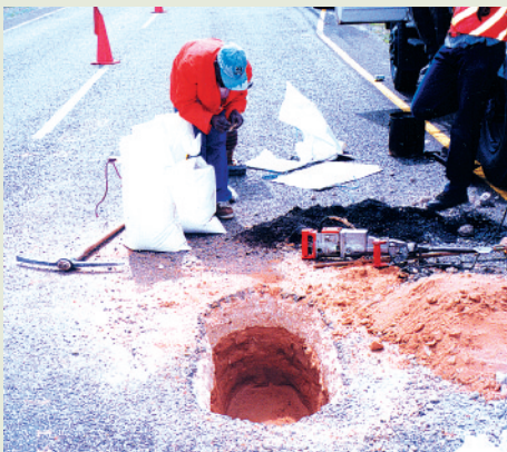
Test pit to check the pavement layers and their characteristics.
