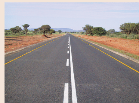
A newly constructed road. Lephephe - Shoshong Road.
