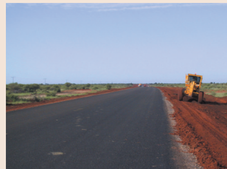
Finalisation of the side drains. Lephephe - Shoshong Road.
