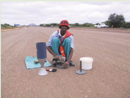
Density control, using the sand replacement method.
