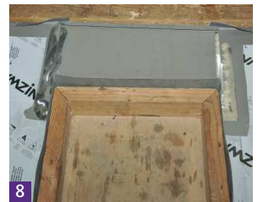
8 Solder back plate into position.
