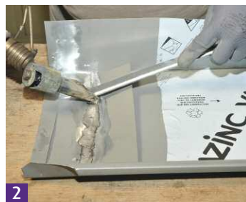
2 Solder welted strip onto panel 150mm below the water check.
