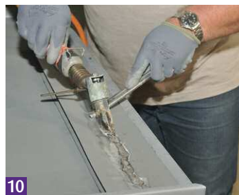
10 Back plate with soldered strip.
