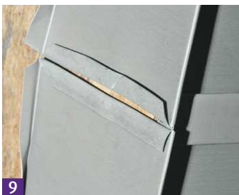
9 Fit adjoining flashing and turn up folds.
