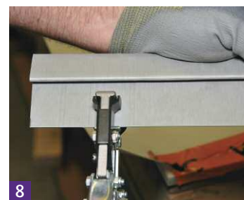
4 The sill is notched back by 50mm. Care must be taken to use a tool that will not leave a tear in the zinc.
