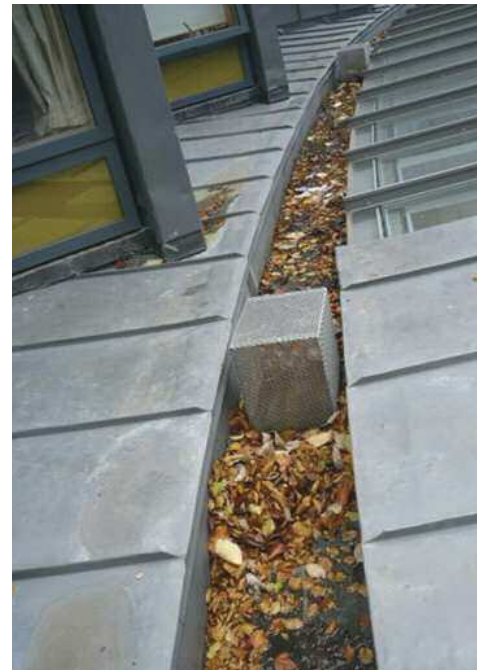
Gutters must be regularly cleaned.
