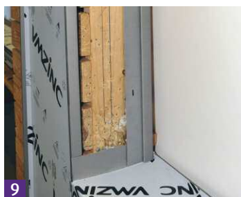
9 The strip is installed.
