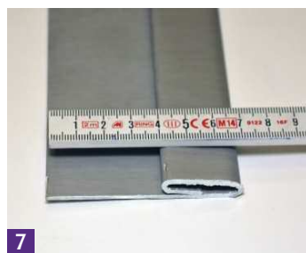
3 The sill is made with a downstand of at least 60mm.
