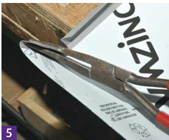
6 Finish fold on panel upstand.
