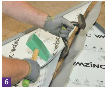
7 The hip batten is installed.
