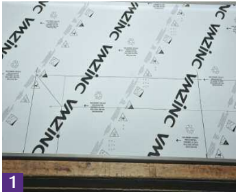
1 Mark out rooflight and include 100mm upstands.
