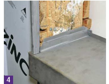
4 The sill (as before) is installed.
