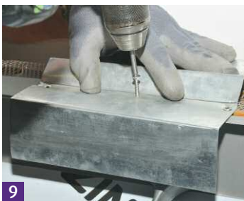
10 Insert ridge flashing.
