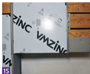
15 The next standing seam panel is installed with sliding clips.
