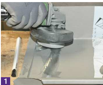
1 Fold 25mm hem on panel and remove patina 150mm further down panel.
