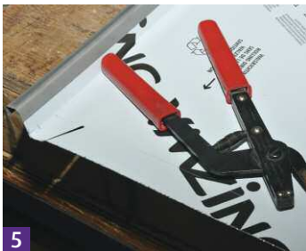
5 The zinc should be cut. Do not use snips that will result in the zinc 'tearing'.
