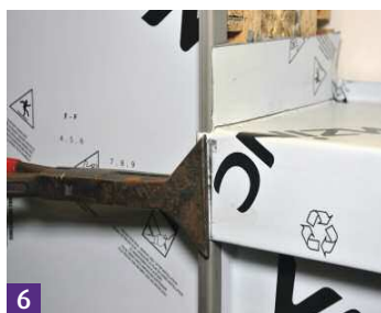
7 The jamb receiver strip is fabricated.
