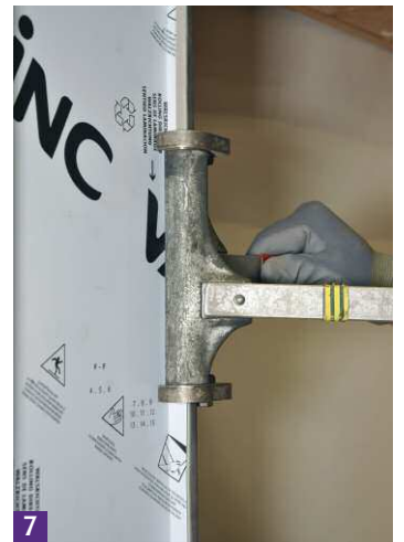
7 Jamb crimped to a single lock.
