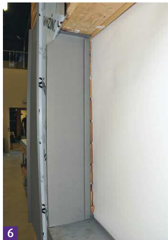
6 Standing seam jamb installed.
