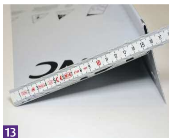
13 The head flashing is made.
