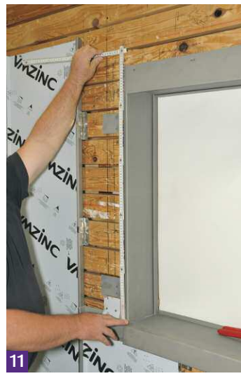
7 Jamb receiver strip installed and jamb measured.
