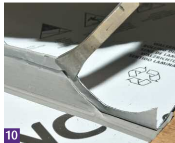
9 Cut the zinc back.
