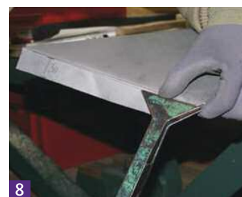
8 The end of the G3 hip is folded back over 30mm.
