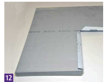
8 Jamb with reveal joint prior to installation.
