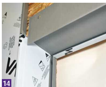
14 The head flashing is fitted using the friction grip and slotted holes for screws.
