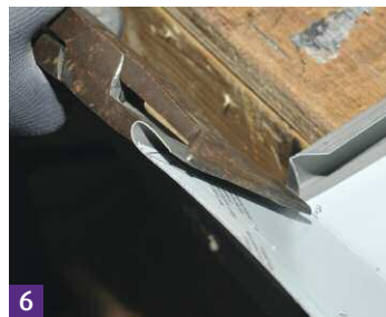
7 Seam panels together.
