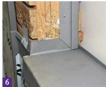
2 A hem for a single welt is formed along with a 90° return for the sill.
