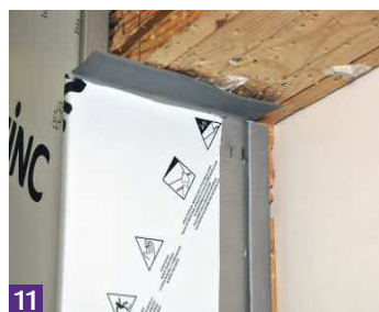
11 The jamb with the friction grip is installed.
