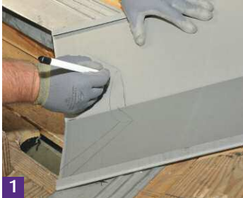
2 Cut the base of the valley back.
