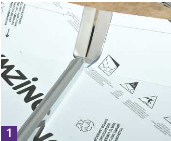
2 Pinch saddle piece into place.
