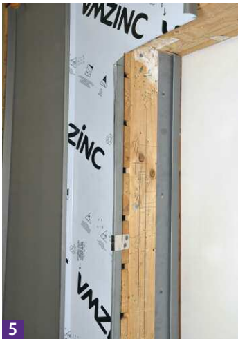
5 Jamb receiver strip is installed.
