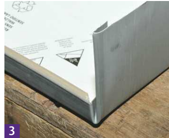
3 Create dog ear fold at bottom of rooflight.
