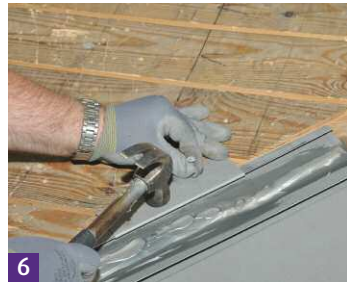
7 Valley ready to receive roofing panels.
