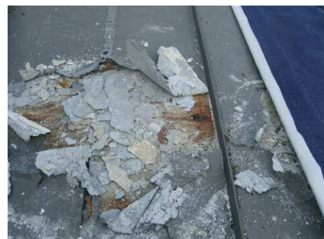
Result of using a hybrid roof.
