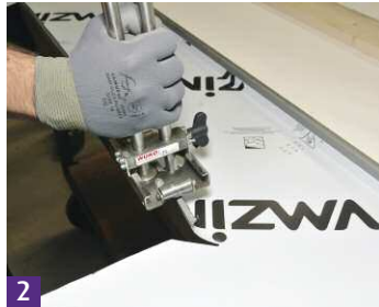
2 An upstand is formed on the panel.
