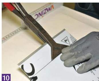
10 A standing seam jamb is made with a 50mm return for the top.
