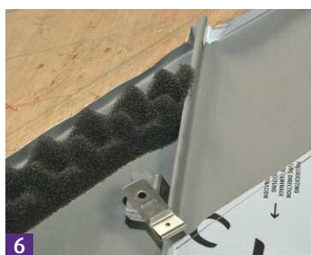
6 The strip is installed (no gaps must be left).
