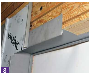
8 Head trim fitted into receiver strip.
