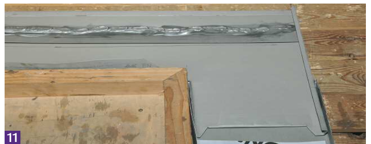
11 Back plate installed as a double welt.
