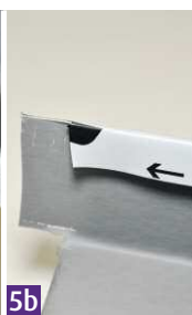
5b The sill downstand is then notched.
