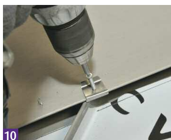
10 The G3 hip is installed into the clip and fixed with a stainless steel screw.
