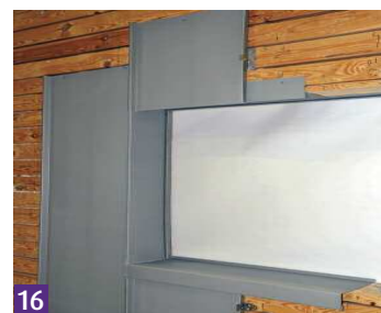
16 Remove plastic film at the end of the job.
