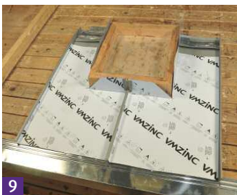
9 Alternative positioning of welted joint.
