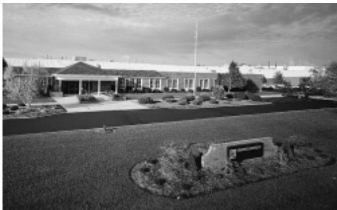
Square D facility in Oxford, Ohio U.S.A. is an ISO 9001 registered busbar trunking manufacturing facility.
