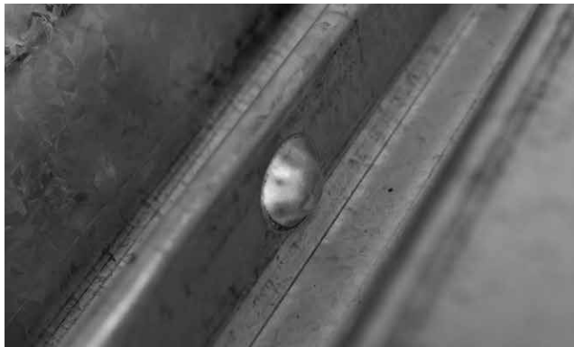
Figure 1.12.2: BUTTON PUNCH SIDE LAPS
