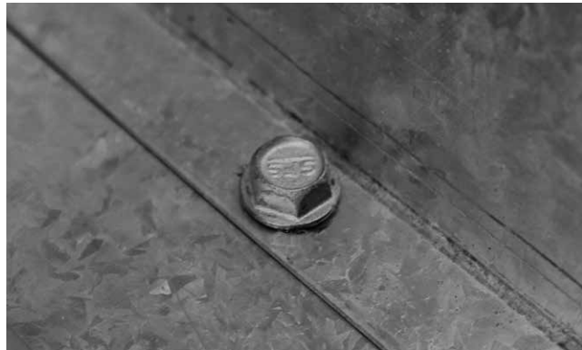
Figure 1.12.3: SIDE SEAM SELF-DRILLING SCREW
