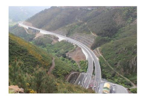
two lanes in each traffic direction, a median barrier, controlled access, wide shoulders and good design characteristics.
