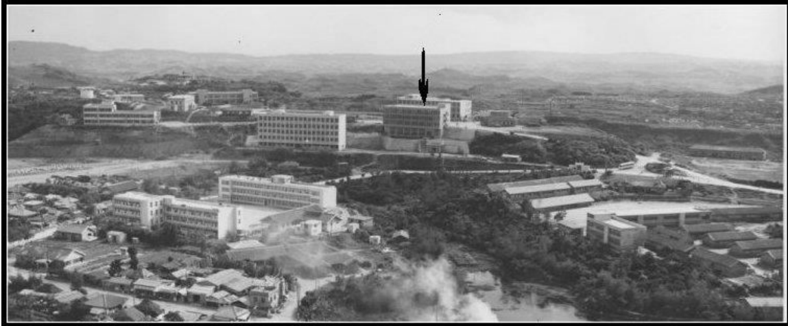
Figure 7. The University of the Ryukyu as it was in the early 1960's. Judo and Kappo classes held in building indicated by arrow.
