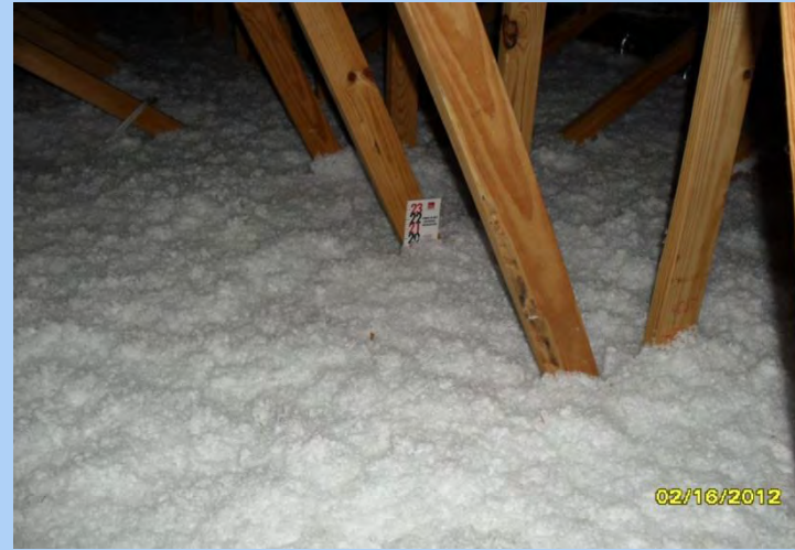
Nice R-50+ Attic Insulation
