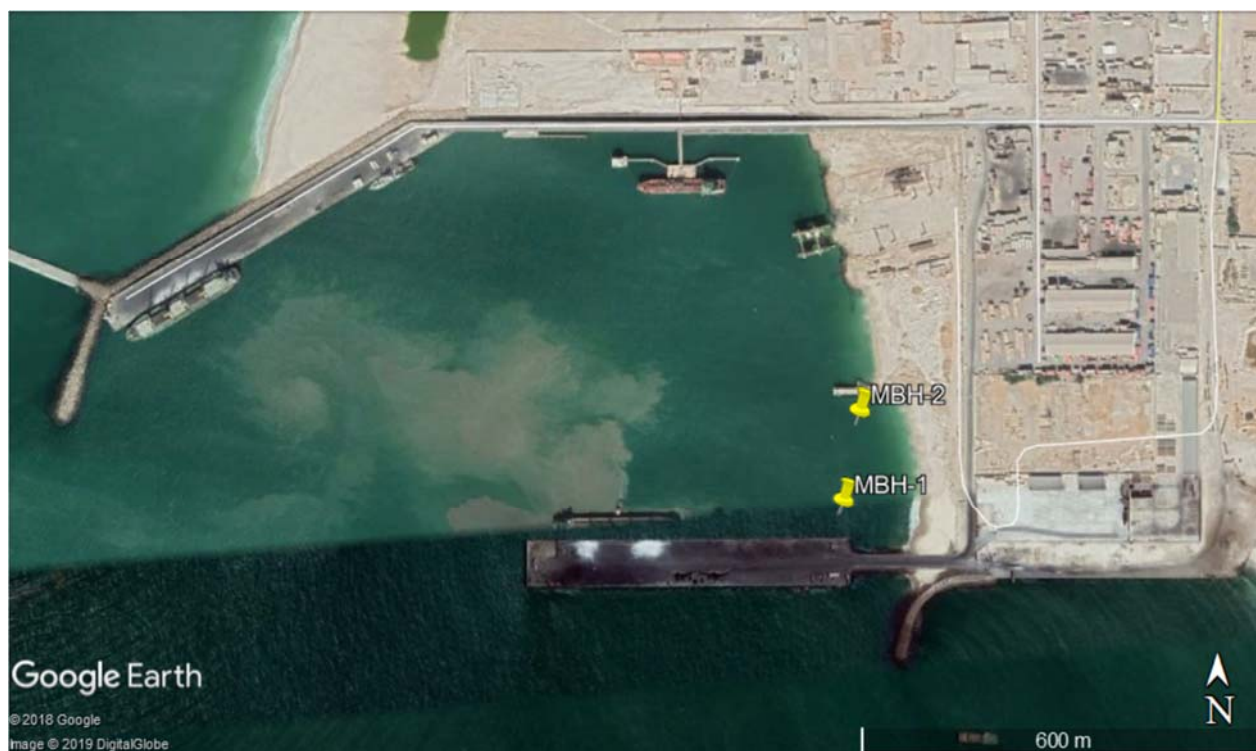
Figure 4-12 Location of vibrocore samples MBH 1 and MBH 2 inside the port basin
