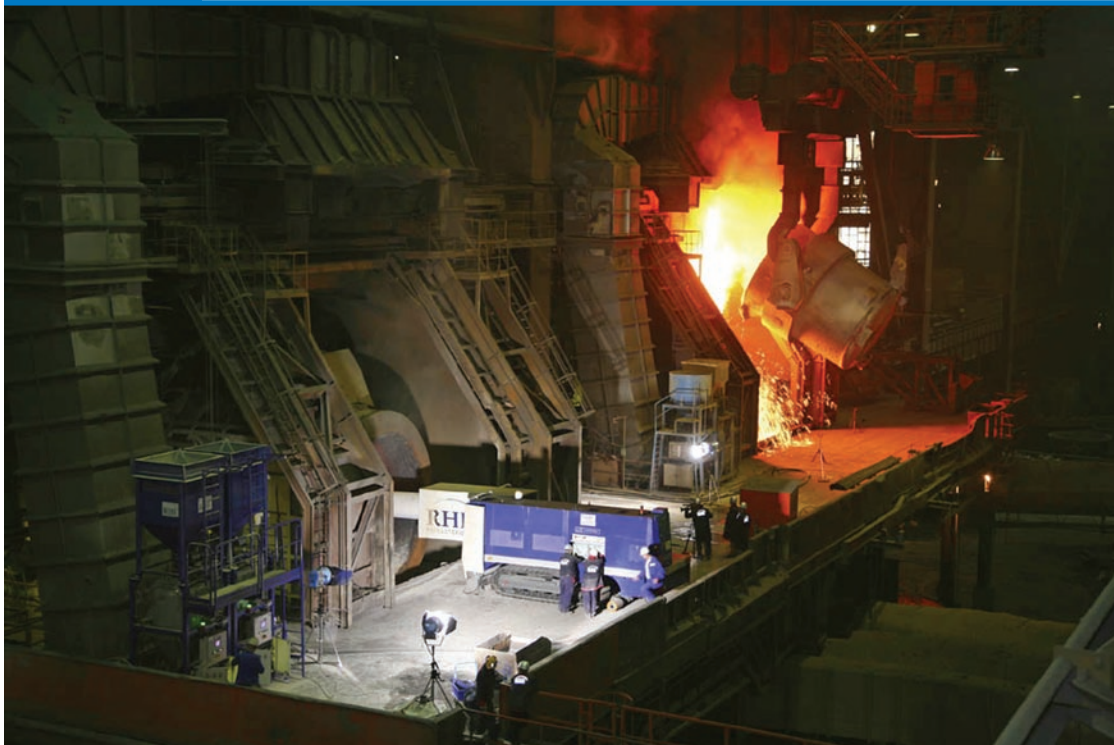
CONREP high-speed gunning system in operation.
