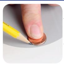
Trace the outline of a penny on the patch material and on the boat. If a larger patch is needed, use a larger item as a template.
