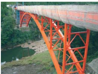
Otobashi Bridge (arch bridge)
