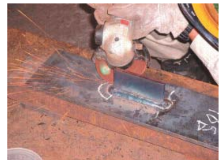
Photo 1 Example of grinder finish of out-of-plane gusset plate weld joint
