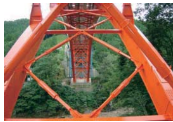
(b) Lateral bracing
