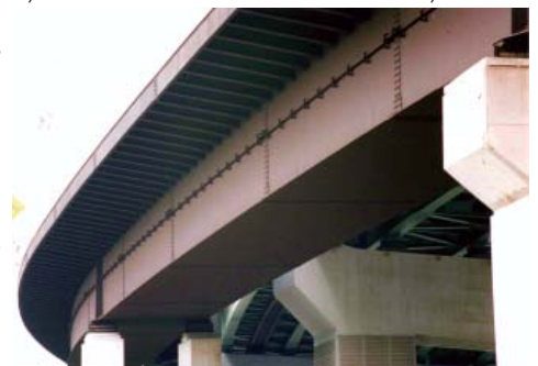
June 2004 (22 years and 6 months after construction)
