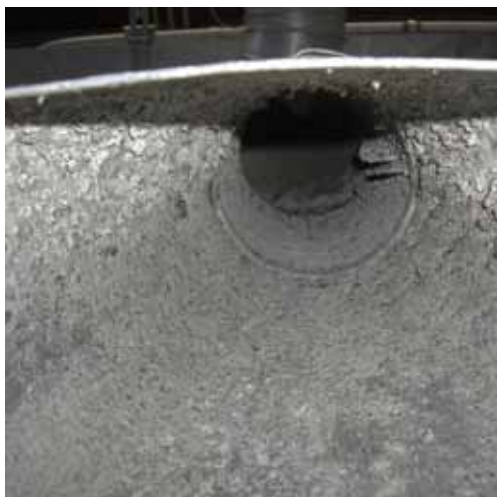
Easily overlooked in a decontamination exercise: the inside of aspirators shown here with a build-up of microbial growth.
