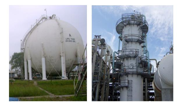
Spherical pressure vessels are usually used as storage tanks, and are recommended for storing large volumes.
