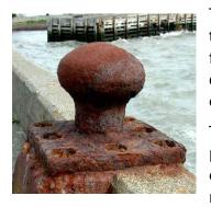
The metal thickness will "wear off" uniformly over time, which is the most common and least dangerous form of corrosion. Other than the detached material, debris, blocking the normal operation of the equipment, this case presents no major complications.
