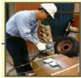
Figure 7: Zinc – Spray (Metallizing)
