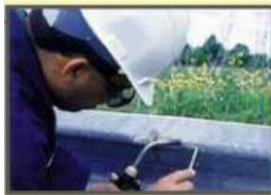
Figure 5: Zinc-Based Solder Technique
