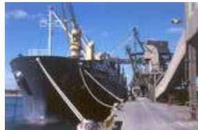
bulk cargo terminal
