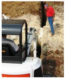
Left: Mini excavator used (narrow bucket) to create trench for AquaBlok placement. Right: Completed antiseep collar around pipe.
