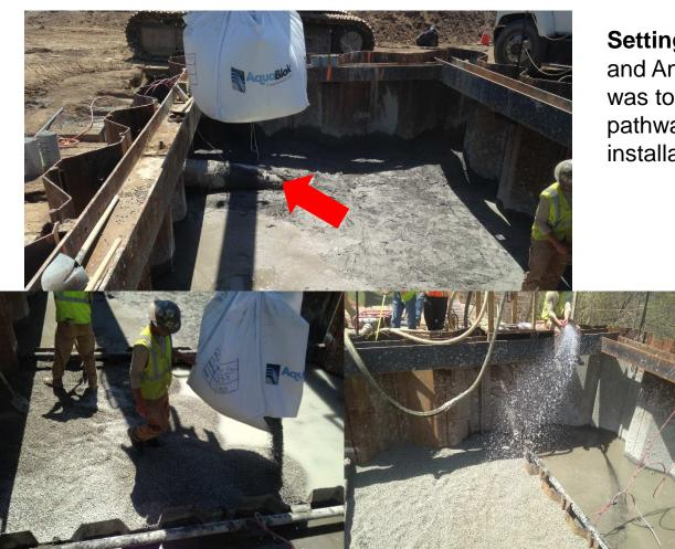
**Setting / Purpose:** Pipeline cap and Anti-Seep Collar. Objective was to cut off site contaminant pathways during excavation and installation of natural gas pipeline.
