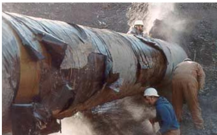
Figure 9.1 – Inspection dig and pipeline repair. (Source: http://www.corrosioncost.com/pdf/gasliquid.pdf )
