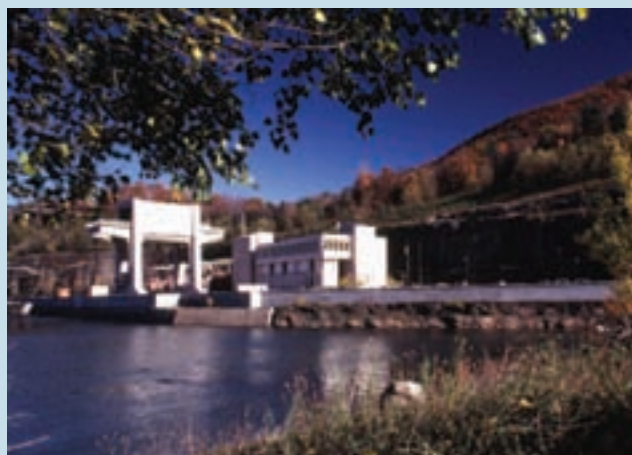
FIGURE 1 Powerhouse at the lower reservoir of the Brown Mountain hydroelectric pumped-storage plant.
