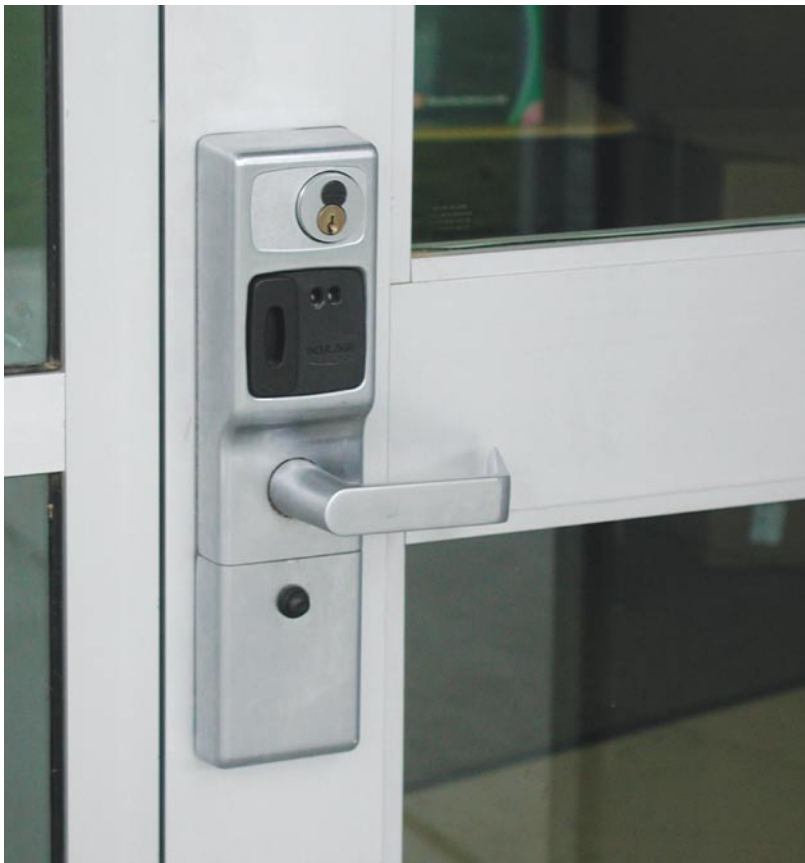
▲ WA993 locks are mounted on aluminum and glass doors as well as conventional steel entrances. ▼ Closeup shows inside of WA993 kit with Von Duprin 98 Series exit device.
