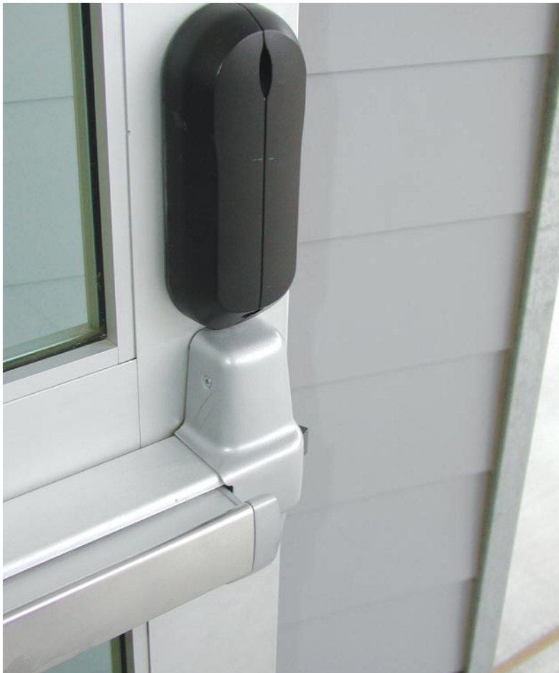
▲ WA993 locks are mounted on aluminum and glass doors as well as conventional steel entrances. ▼ Closeup shows inside of WA993 kit with Von Duprin 98 Series exit device.
