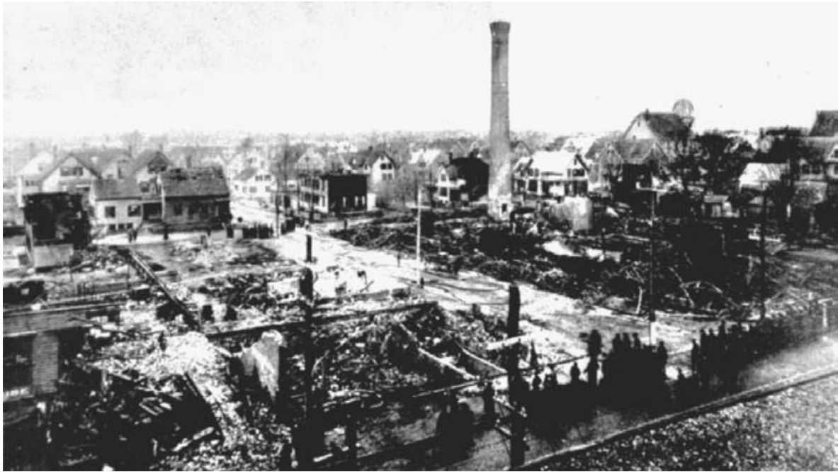
Figure 1.2 Shoe factory after the boiler explosion of March 20, 1905, which led to the adoption of many state boiler codes and the ASME Boiler and Pressure Vessel Code . (Courtesy of The Hartford Steam Boiler Inspection and Insurance Company .)
