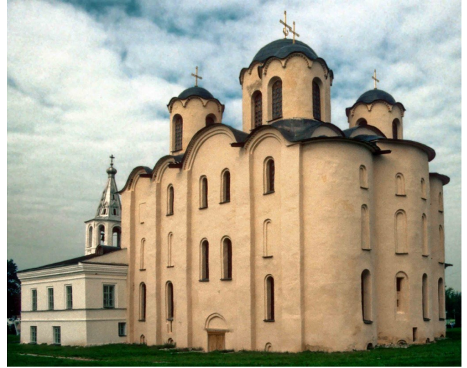
Fig. 5. The Church of St. Nicholas in the prince’s court, here restored to its original five-domed appearance. View from the southeast. The porch on the left was added in modern times. (Photo courtesy of Daniel C. Waugh)
