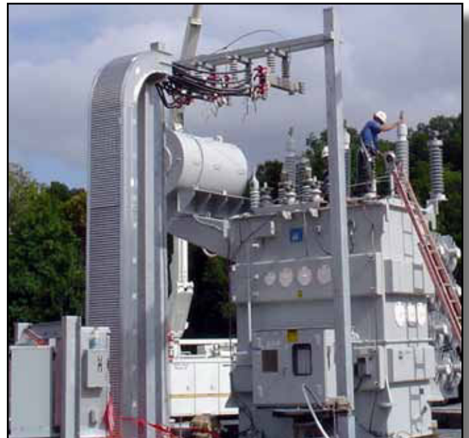
MP HUSKY 4000Amp, 5kV Cable Bus system with open air termination to GSU transformer.
