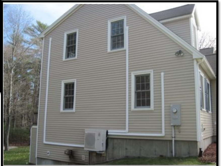
Below: Outdoor conduit shown running from the outdoor unit to three indoor units.
