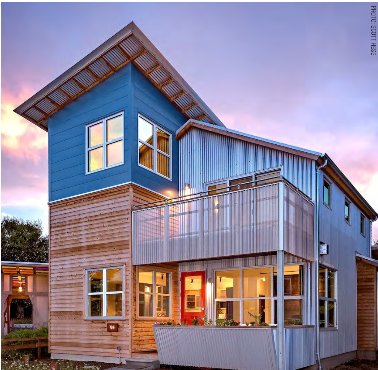
Bright colors contrast with the subtler palette of cedar and metal. On the commons building, a local artist used colored lime and frescoing techniques on cementitious boards to create vibrant pattern. It's offset by burnt cedar boards done in the Japanese Shou Sugi Ban technique.
