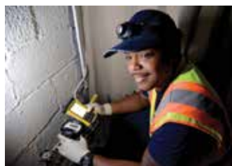
Meter upgrades in Bayonne reduce non-revenue water for the city
