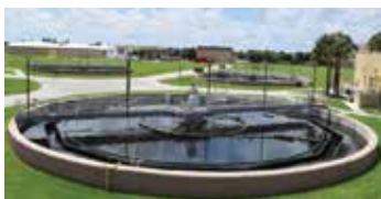
Palm Beach County Aeration Facility
