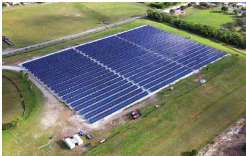
Solar farm atop Lake Worth landfill
