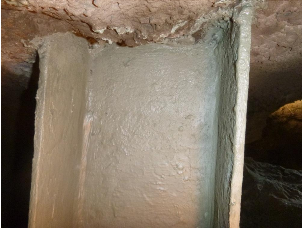
Figure 35. Field application of zinc rich organic primer
