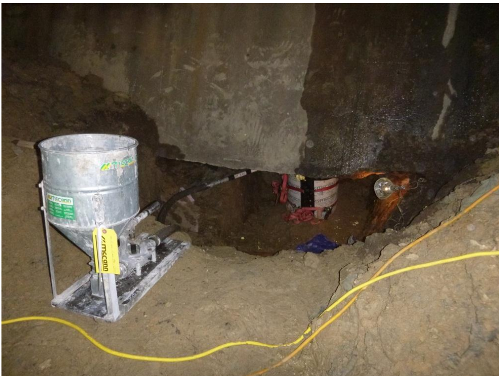
Figure 38. Filling of grout form using manual grout pump
