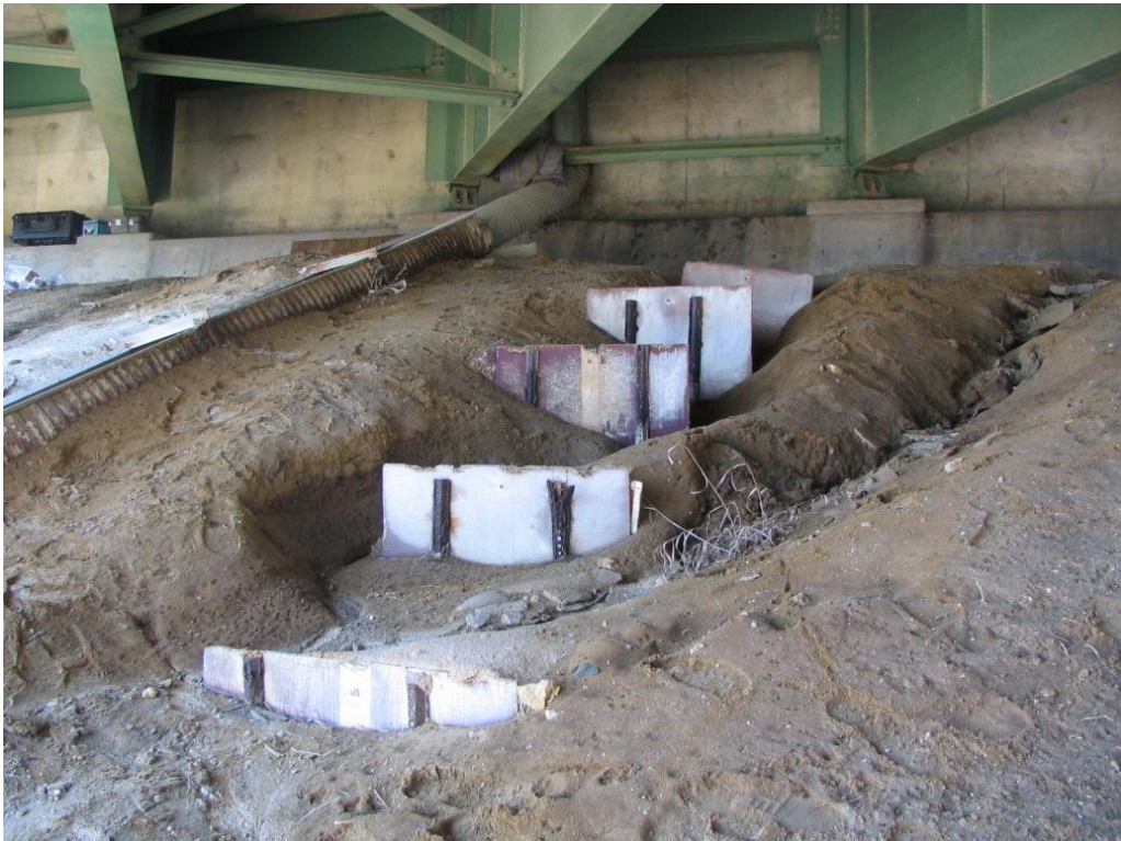
Figure 2. Staked plywood sheets for erosion control
