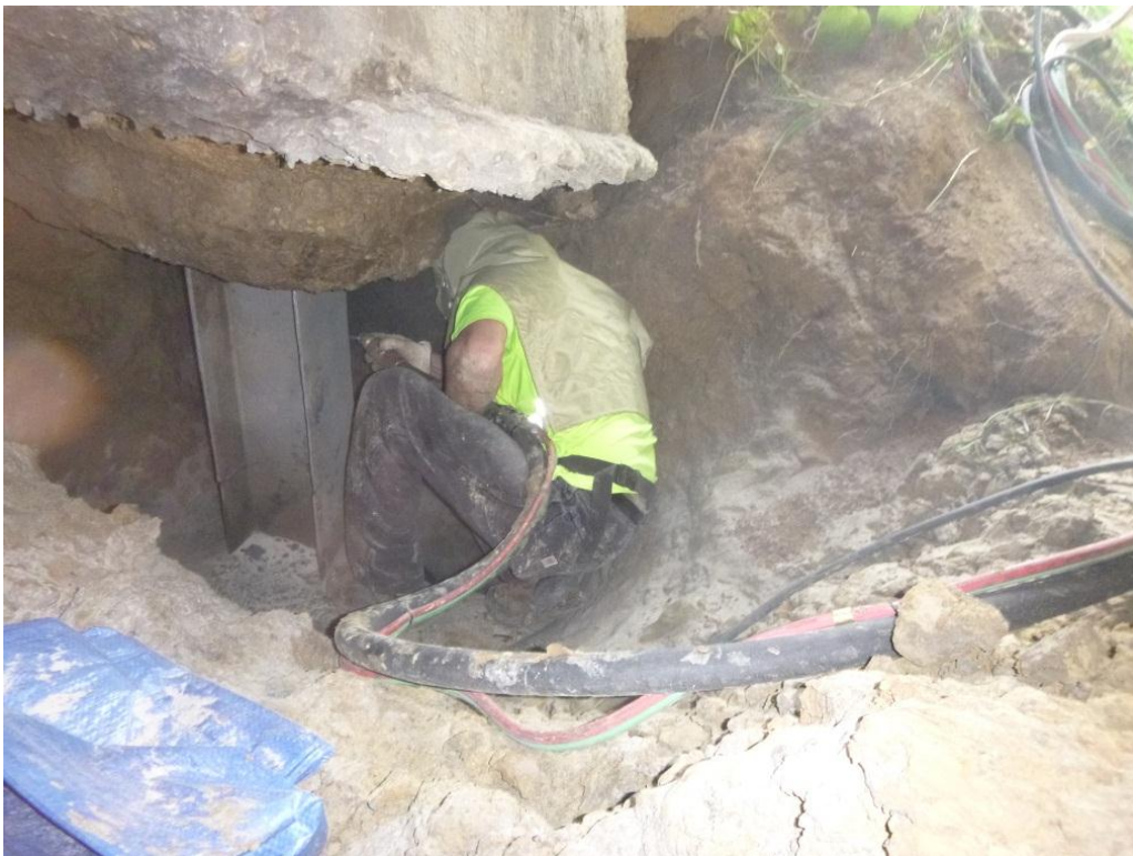
Figure 28. Abrasive blast cleaning of Pile 1
