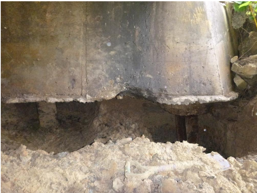
Figure 26. Excavations at Piles 1 and 2
