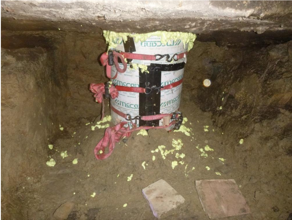
Figure 37. Completed form for formed grout encapsulation
