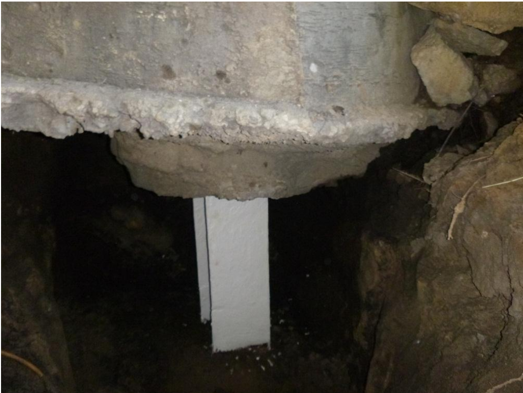
Figure 34. Field application of polyester glass flake coating
