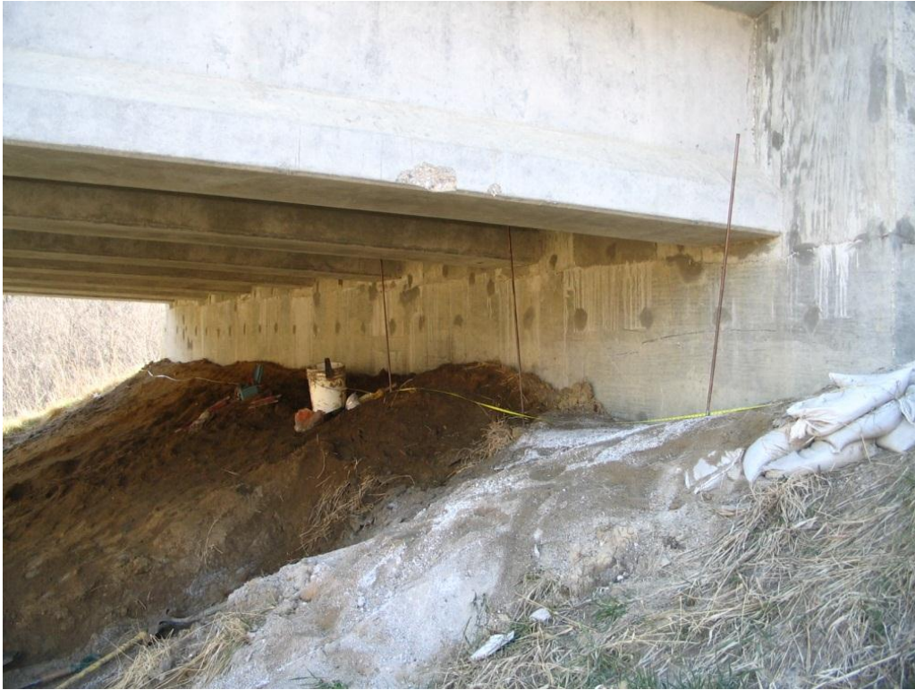
Figure 3. Erosion repair using grout material
