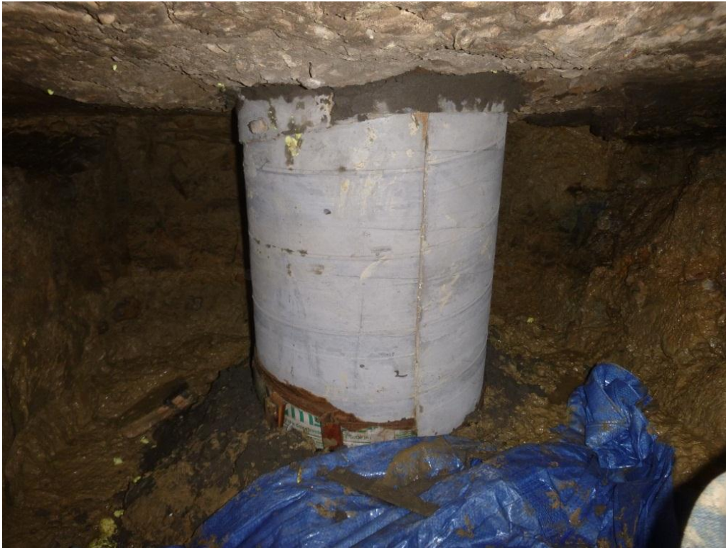
Figure 39. Completed formed grout encapsulation
