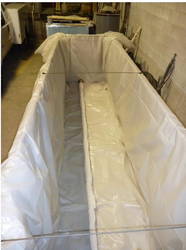
Figure 44. Perforated drain and poly sheet barrier.
