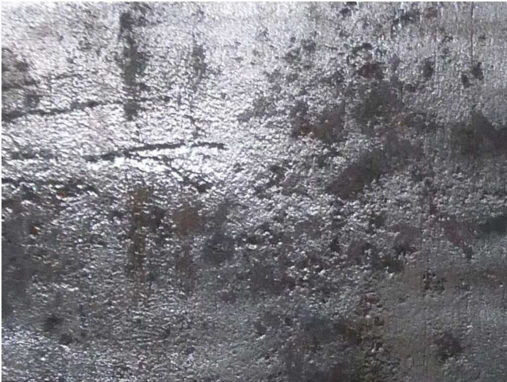
Figure 32. Typical prepared surface using the MBX Bristle Blaster
