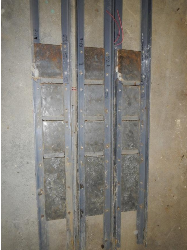
Figure 60. Piles after cleaning with wire brush
