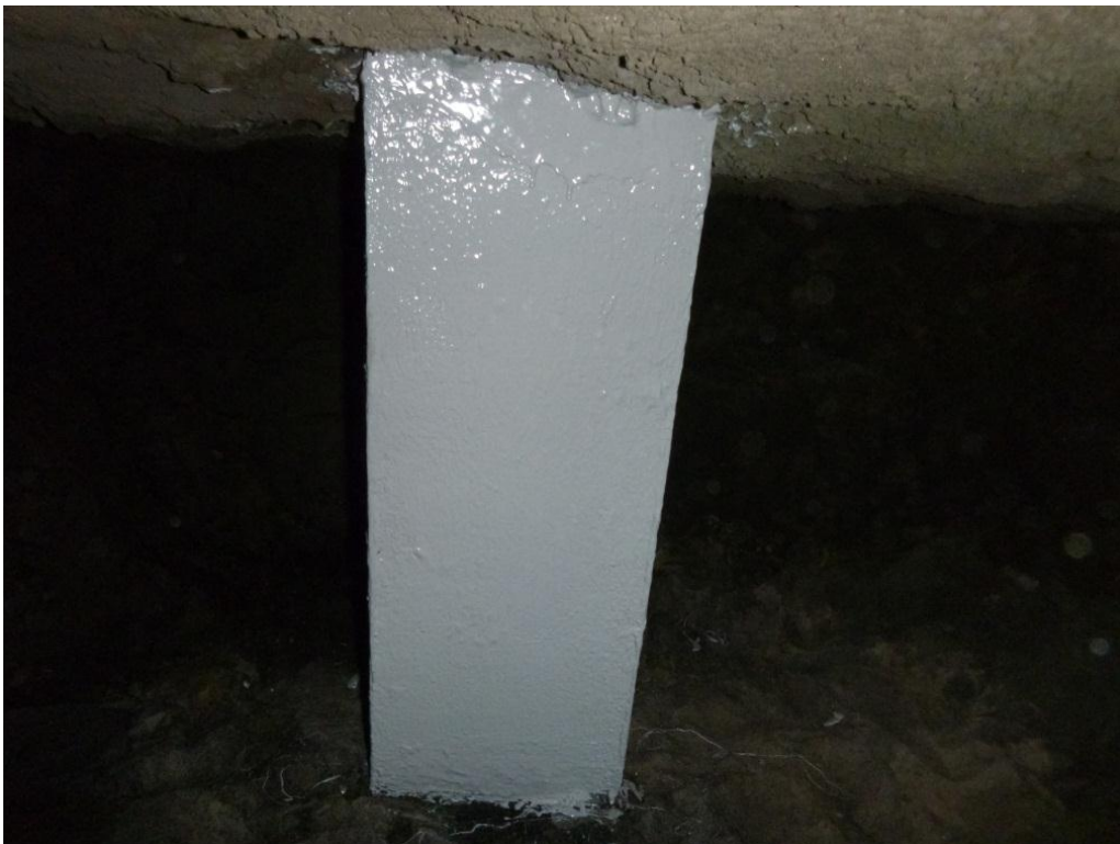
Figure 36. Field application of epoxy top coat
