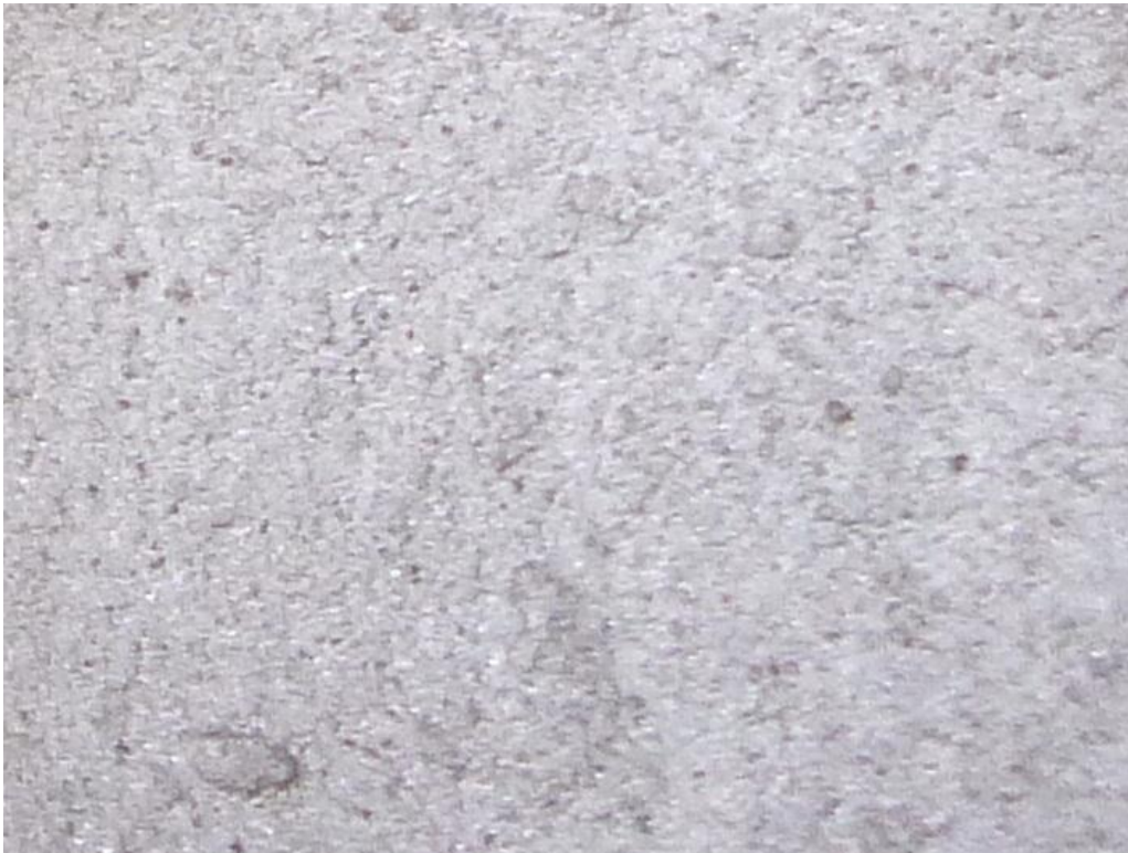
Figure 31. Typical abrasive blast cleaned surface at relatively easy to reach area of pile
