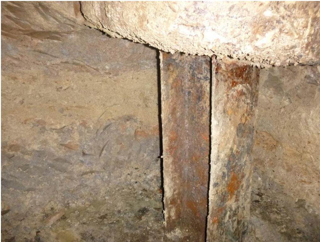
Figure 27. Pile 1 after mechanical removal of soil from pile surfaces
