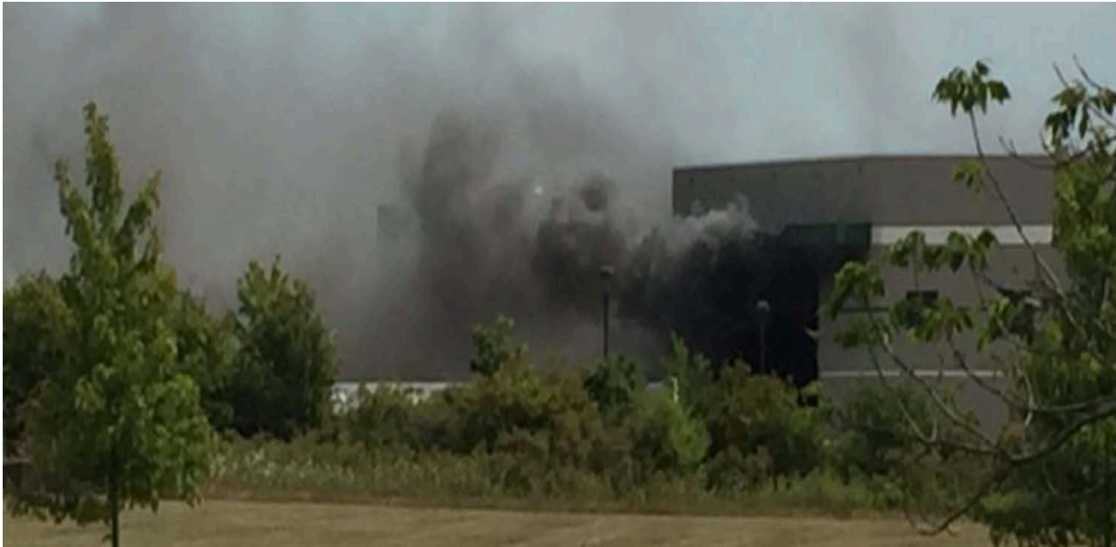
Figure 11 Fire involving Li-ion ESS inside S&C Electric Manufacturing Facility
