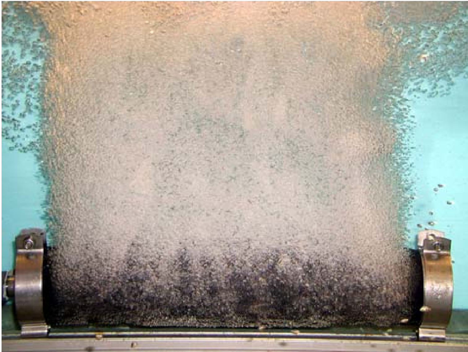
Diffused Air System
