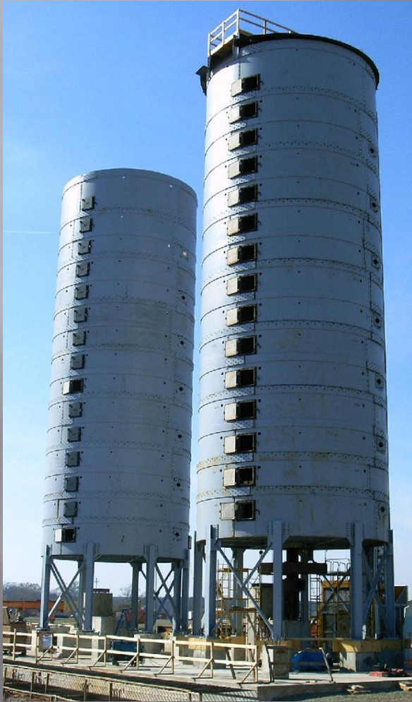
Two large MHFs under construction
