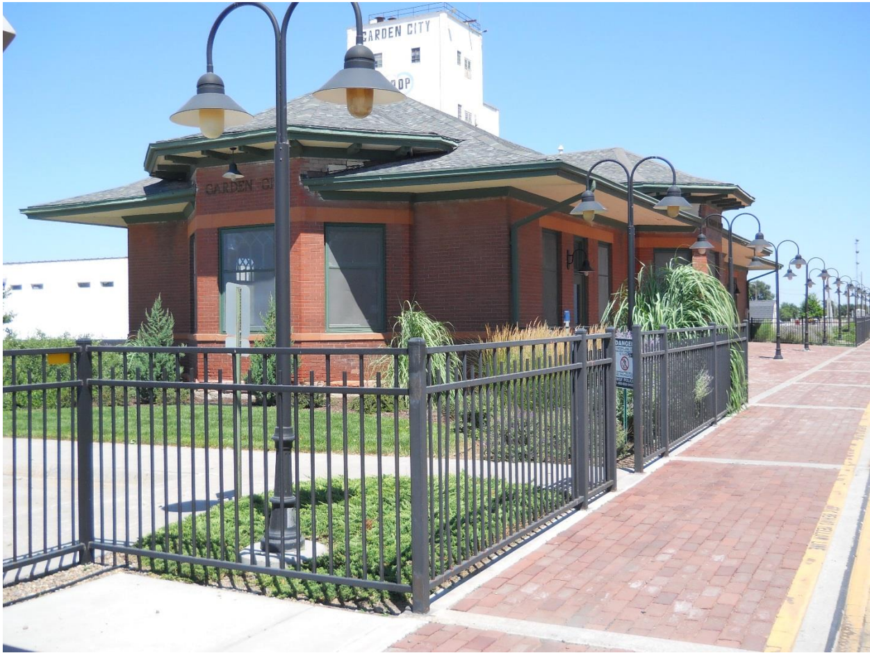
Figure 2.26: Garden City Station
