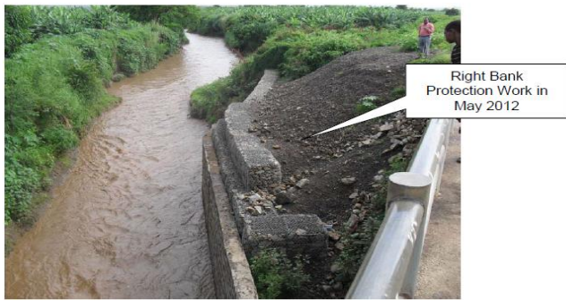
Figure 2.3. Bank with embankment protection work in May 2012.
