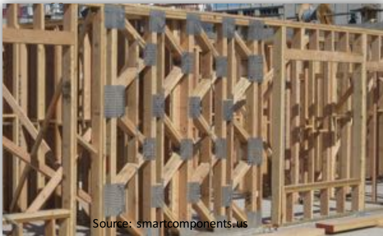
Proprietary Trussed Shear
