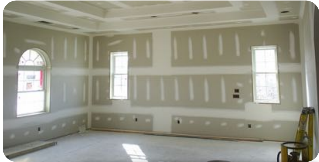
Gypsum Shear Walls
