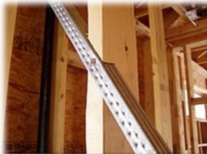
Bracing installed in a saw kerf
