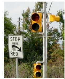
Figure 6-3: Ramp Meter Signals
