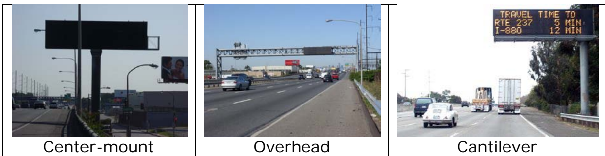
Figure 3-7: DMS Structure Types
