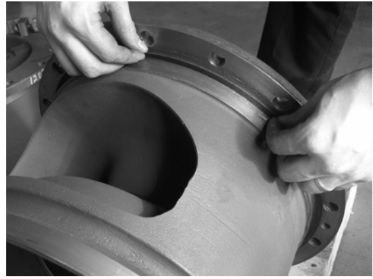
Figure 38: Installing the Gasket on the Coverplate
