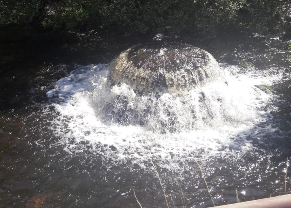
Figure 6.4: Photo showing outfall of compensation flow culvert
