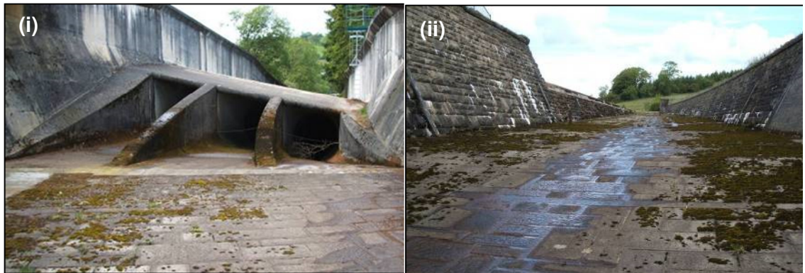
Figure 5-1 Stocks reservoir spillway photographs
