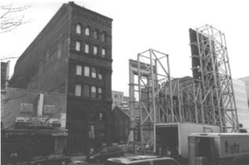
A preservation easement donated to the National Trust for Historic Preservation on the late 19th Century National Union building saved it from the fate of its neighbor. While the National Union building, on the left, is mostly intact, the historic buildings on the right retained only their street facades (photo courtesy of the National Trust for Historic Preservation, Washington, DC).
