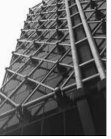
Structural tubes, filled with water, used as an external fire prevention system.
