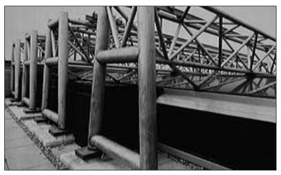
Stainless steel trusses (20 meters) for bracing and end frames for skylight supports.
