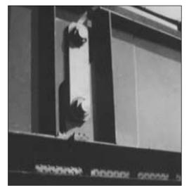
The Minnesota Department of Transportation replaced conventional low alloy steel with stainless steel hinge pins and hangers on the Blatnik Bridge in Duluth, Minnesota.
