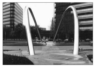
Arches, strut light covers and traffic signal poles (not in photo) were fabricated from 316L Stainless steel by the Offenhauser Company. The project is in the Galleria area in Houston.
