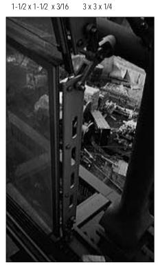
Complex stainless steel investment casting connecting the tubular structure with the glass wall.
