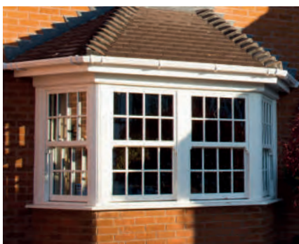
Bay window with vertical sliding sash windows
