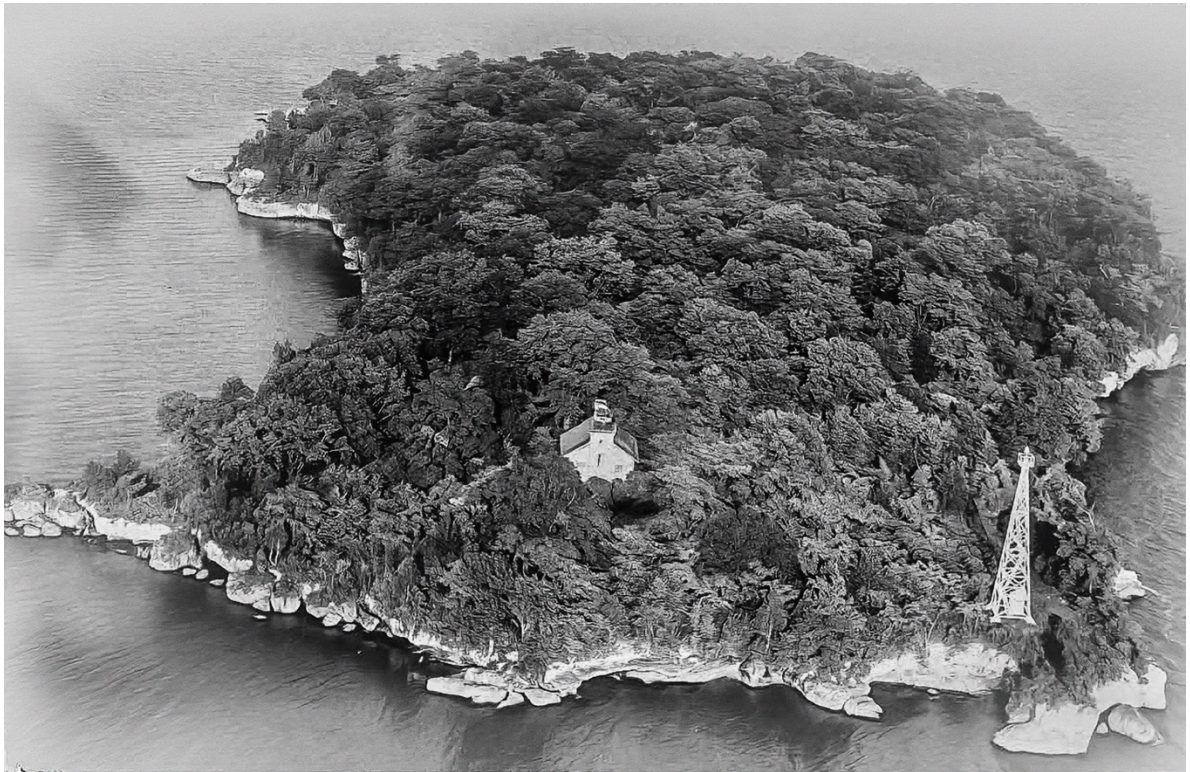
Figure 22: 1954 Aerial View showing the old lighthouse and new light tower
