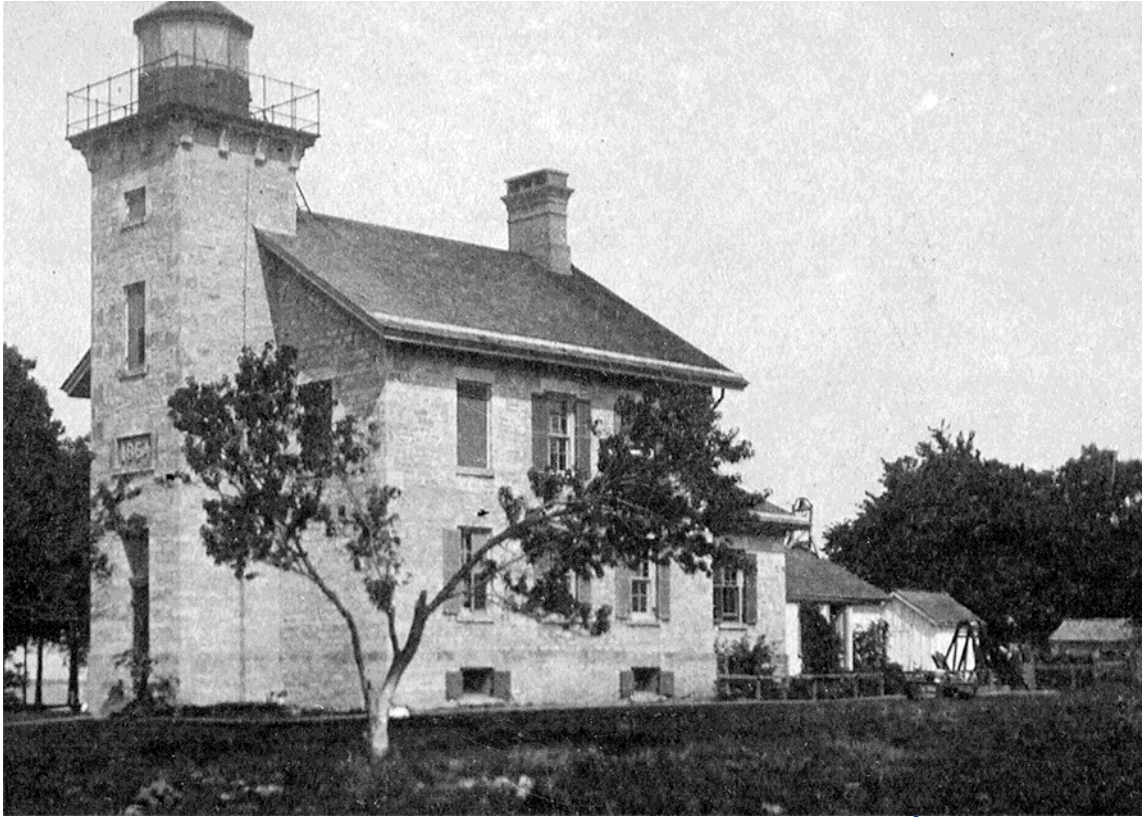
Figure 9: Green Island Lighthouse, A Second Photo from Around 1920 5
