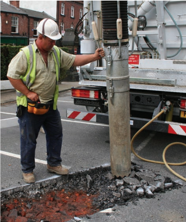
Suction excavator (courtesy of TT-UK Ltd.)
