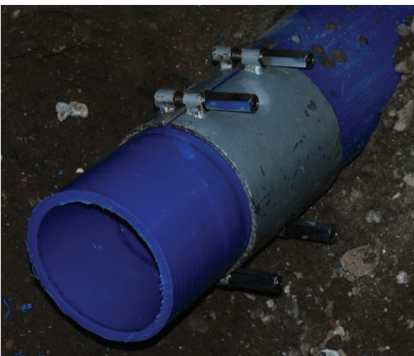
Coiled pipe being re-rounded
