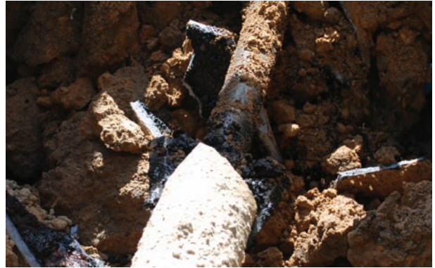
Pipe bursting in progress
