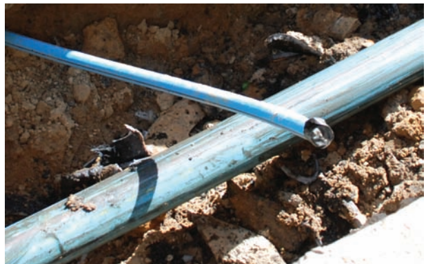
New pipe pulled into position
