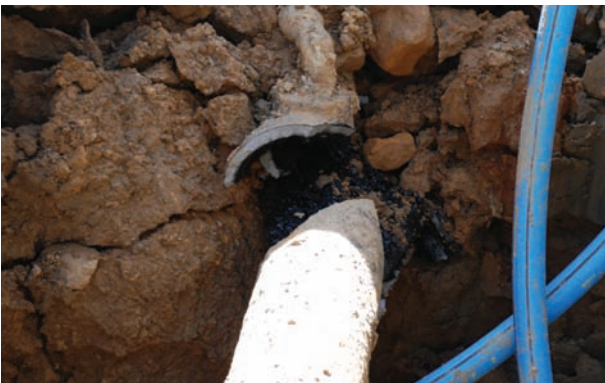
Entry of bursting head to service trench
