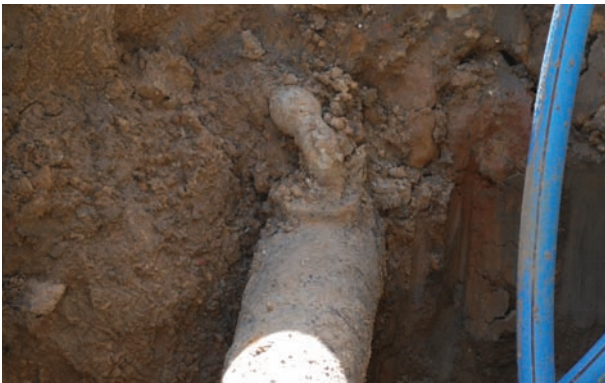
Original pipe in service trench
