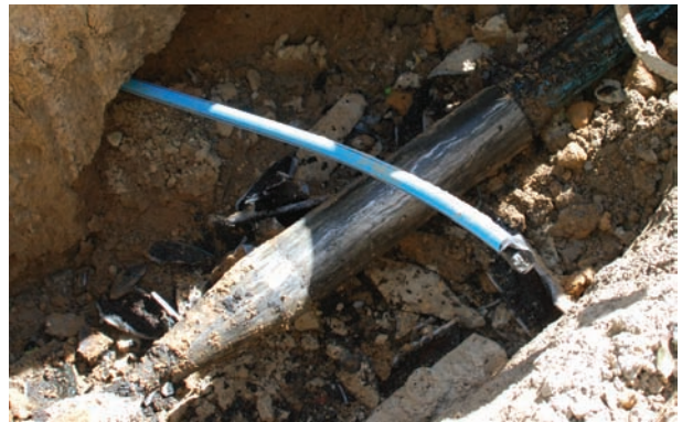
Exit of bursting head from service trench
