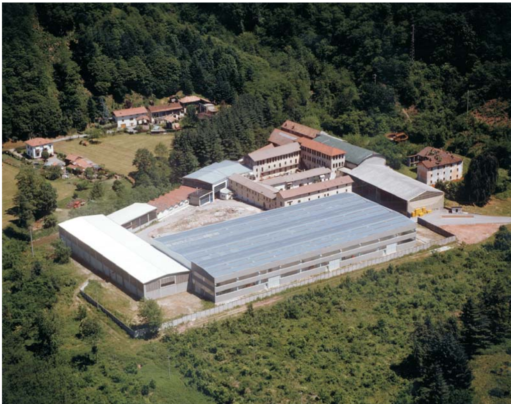
second location in Borgosesia loc. Baraggione - storage - gamma-ray bunker for radiographic tests
