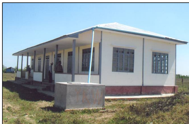
School reconstructed by MoE with rain water storage features
