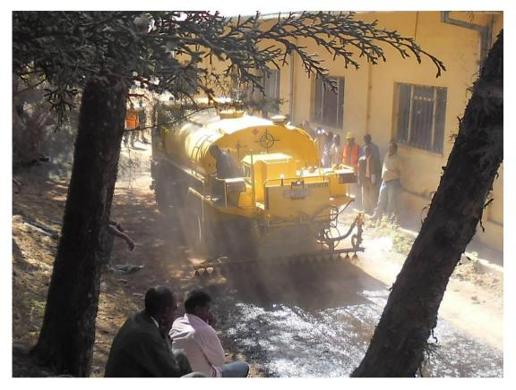
Figure 3 Carrying out the longitudinal spray rate test
